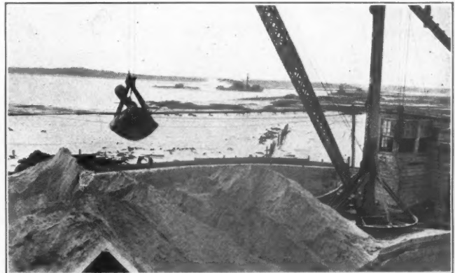
Fine Sand Settling Basin of Concrete and Unloading Hoist
